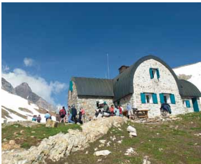
Refuge de Baysse - Pyrénées - © FFCAM
