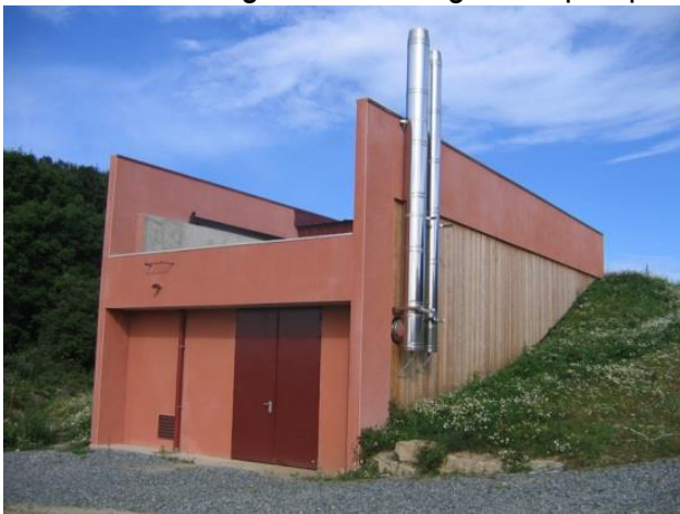
Chaufferie collective – Izeron – 38
